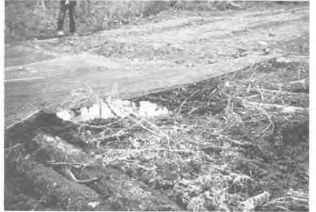
Figure 18. On haul roads rutting occurs unless granular thickness reduces subgrade stress to four times clay surface shearing strength ( 4c_u , i.e., 0.67 \times CBR ).
