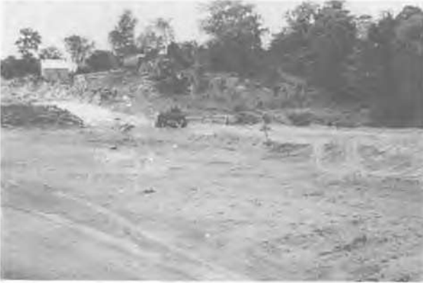
Figure 15. Construction to thickness. Note grade stakes settle with construction.
