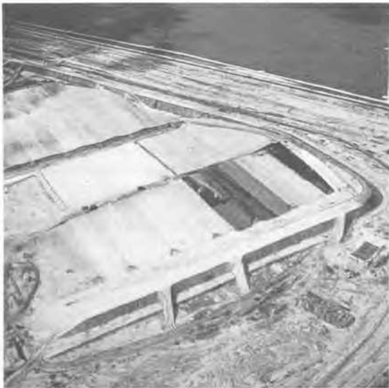
Figure 3. Construction of edge dam and technical barrier.
