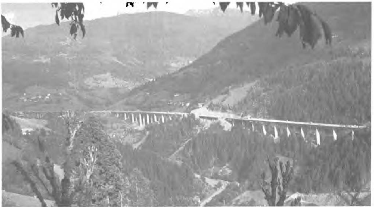
Fig. 10: Partial view of an Alpine highway in Austria, running on steep, slide-prone slopes in a seismic area (up to 10° MS).
