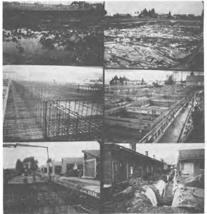
Fig.3. Details of spread hinge-tied foundation construction
