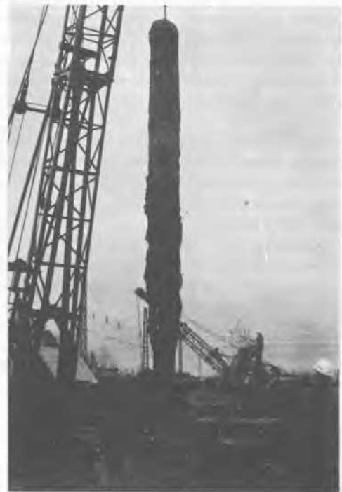
Figure 7. Recovery of a Test Pile
