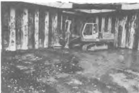
Fig. 12 Uncovered soilcrete-slab a) investigation shaft in field 1 b) milling machine grinding the soilcrete-slab surface
