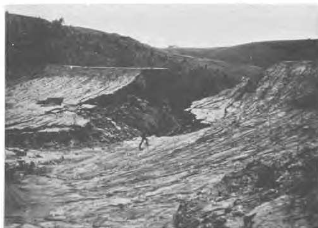
Fig.2 Failure of earth dam.
