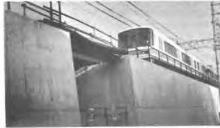
Plate.1 View of the train running on the geosynthetic-reinforced soil bridge abutments
