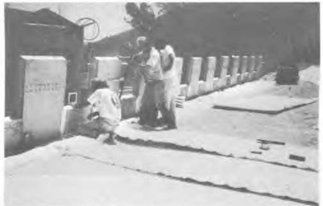
Fig. 1. GeoMesh Reinforced Soil Retaining Wall
