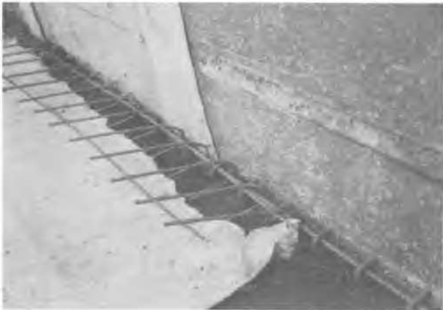
Fig. 2. Connection between GeoMesh and the wall facing.
