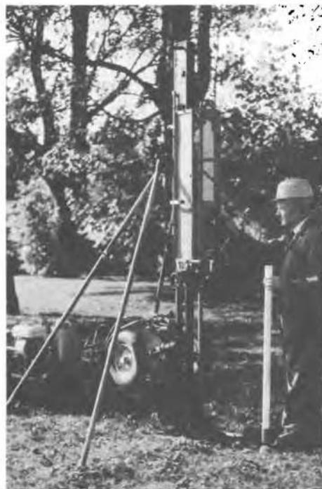
Figure 1. Ram Sound Equipment with standard rod and point. Operator holding standpipe installation.
