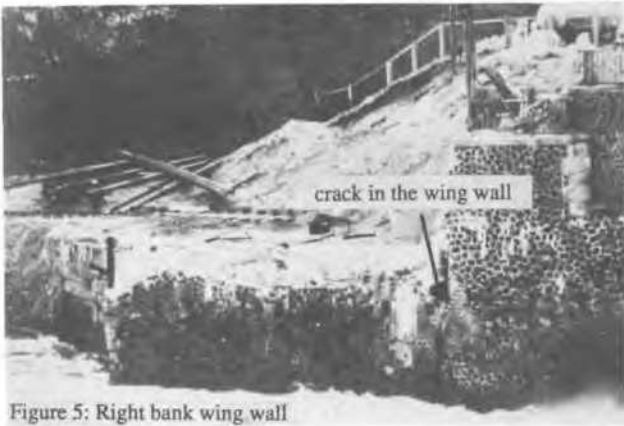
Figure 5: Right bank wing wall
