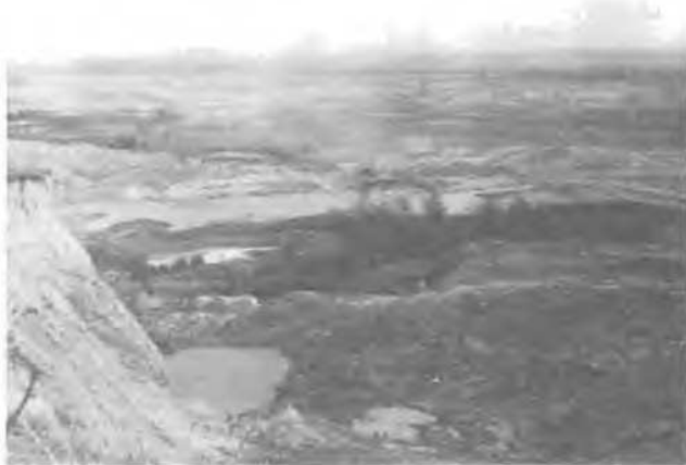
Figure 2. Border of the landslide
