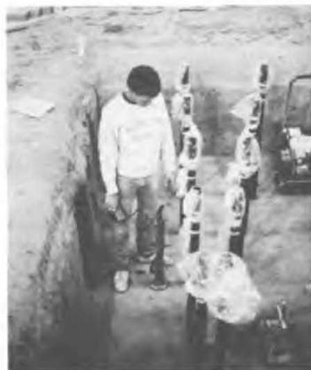
Fig. 3 Piles During Installation Stage
