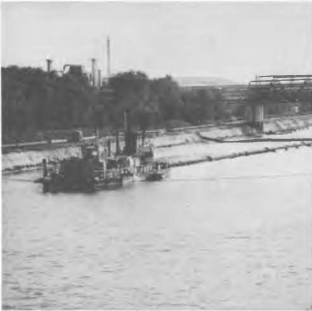
Fig. 9. Suction-cutter dredge in operation enlarging the canal cross section
