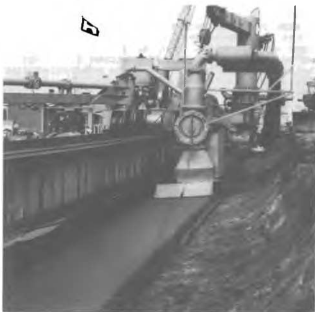
Fig. 7. Laying device with mouthpiece for laying the sealing layer.
