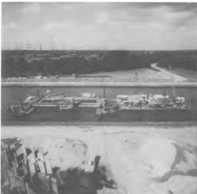
Fig. 6. Laying unit consisting of preparation and laying boat.
