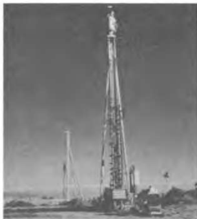
Figure 3. SMW Two-Auger Machines
