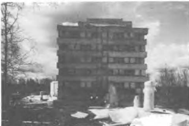
Figure 16. Counterbalance weight construction for loading of the long piles.
