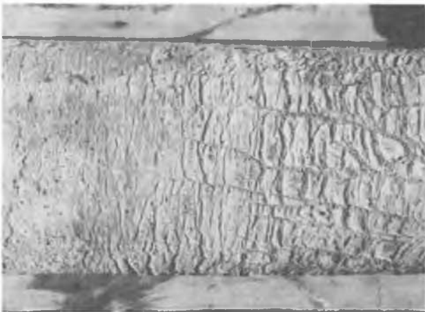
Figure 23. The reticular cryogenic structure observed on the surfaces of the piles.
