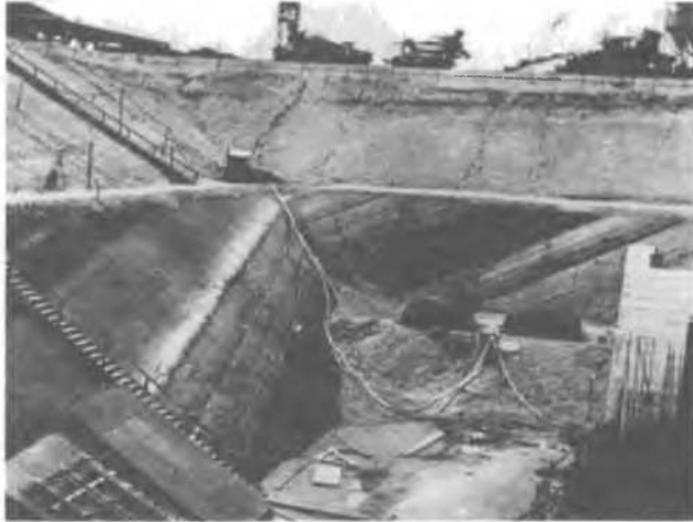
Figure 3. South-western corner of the foundation pit.
