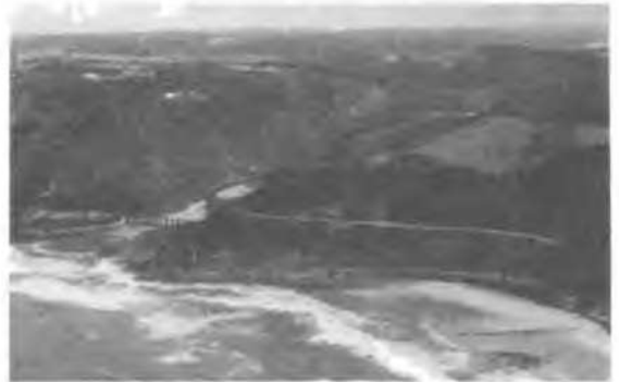
Fig 2 : Aerial photograph of the road section
