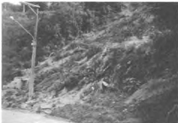
Figure 3. Thick silty clayey coluvial soils with low angle.
