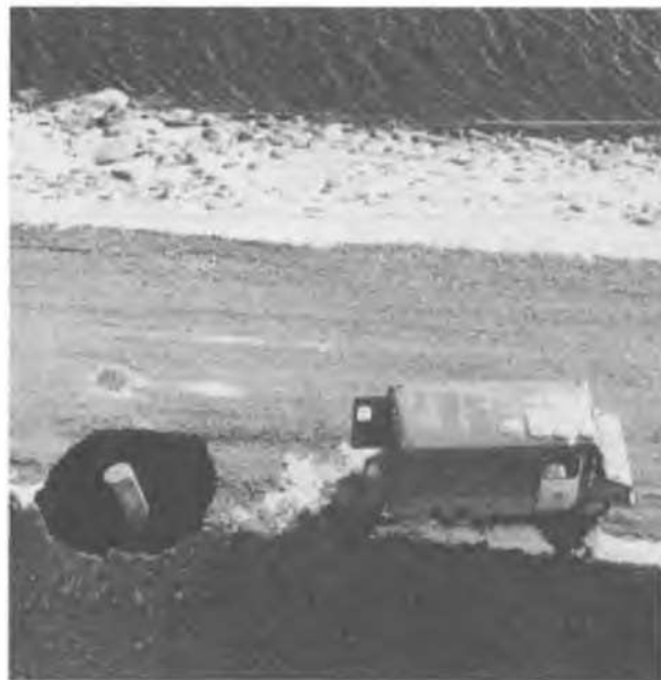
Figure 1. QA-8 dyke - Crest sinkhole and raiser pipe.
