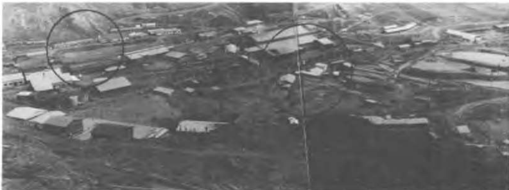
Figure 1. General view of the site plant area and location of the damaged structures
