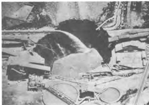
FIG. 5: ACTIVE WATER TABLE - SINKHOLE WHICH ENGULFED THE WEST DRIEFONTEIN CRUSHER PLANT - 1962
