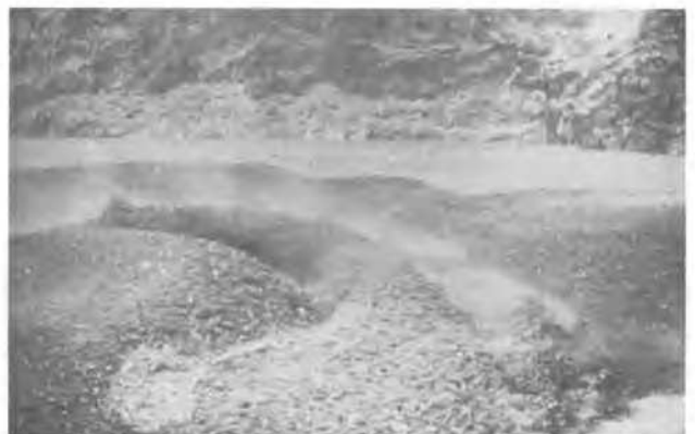
Figs 3a), 3b): Views of debris waves emerging from Nala and spreading across dam.
