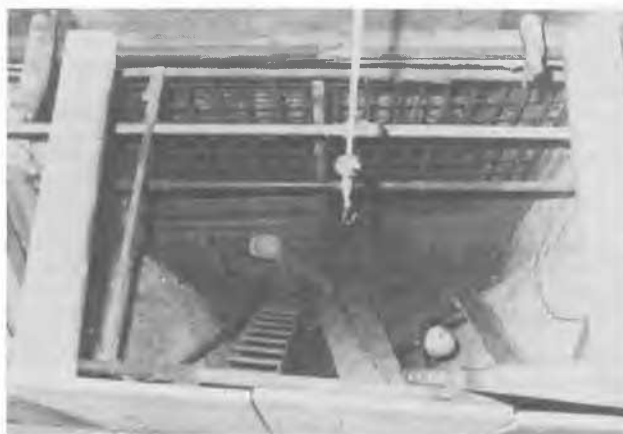
Fig. 8 - Construction of a pier foundation panel inside a frozen soil cylinder.
