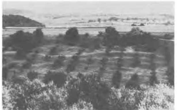
Fig.1 Typical creeping slope
