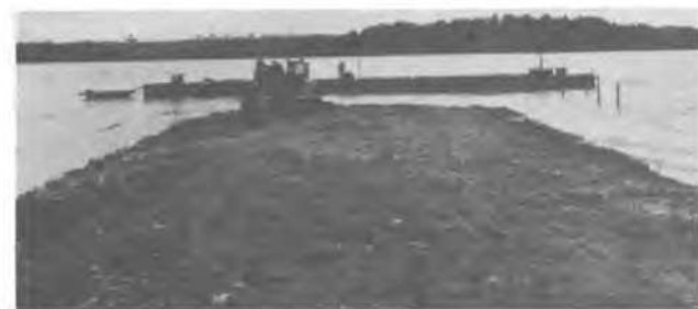
Figures 11 and 12. Embankment under construction
