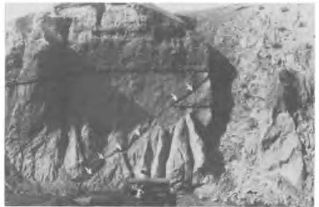
Fig. 2 Faulting in terrace deposits near Kalabagh Fault
