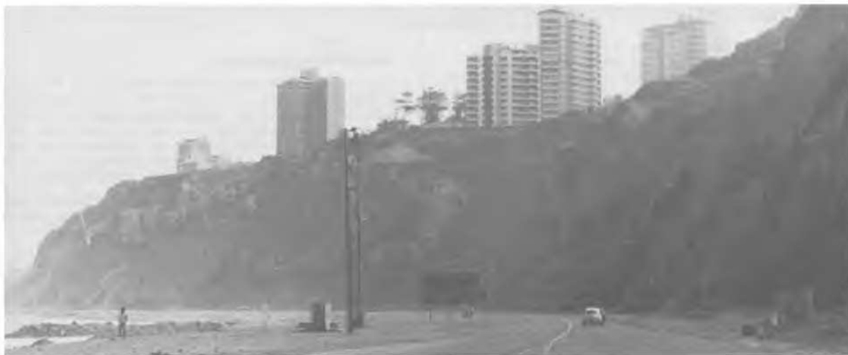
Fig. 1- General view of the actual conditions of the cliffs
