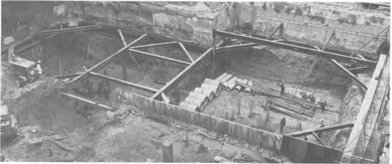
Figure 1(b) Bracing Grid Temporarily Supporting Diaphragm Wall
