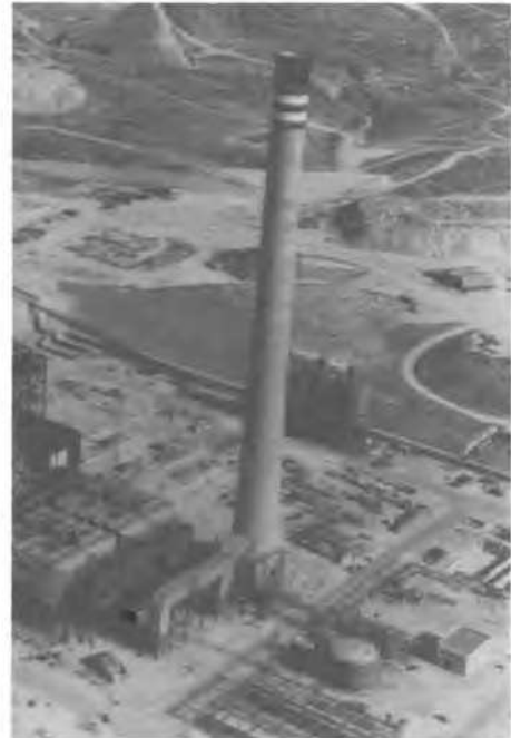
Fig. 1.- View of the 200 m high chimney
