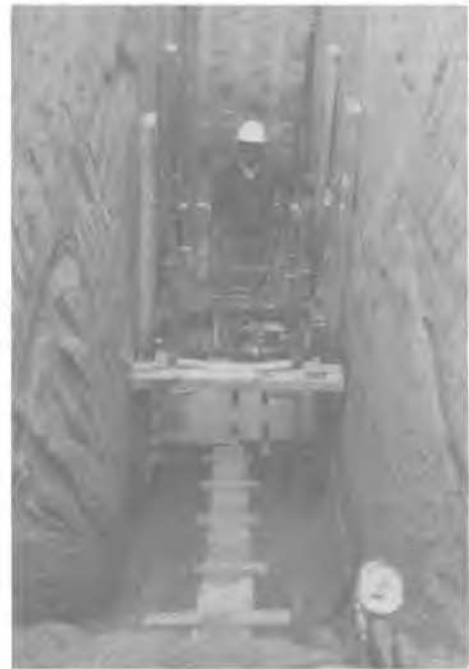
Fig. 6.- Horizontal plate deformability test Ø 60 cm
