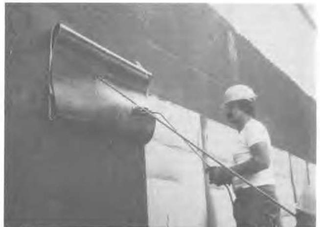
Fig. 3 Application of the bituminous slip-layer.
