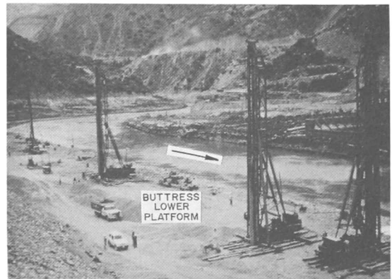
Fig.10 Sediment Treatment - Franki and Vibroreplacement Rigs
