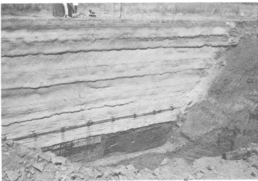
FIG. 3 A View of the Excavation Site
