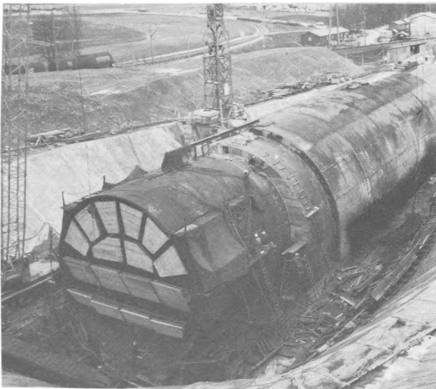
Fig. 3 Circular shield with breasting doors East portal
