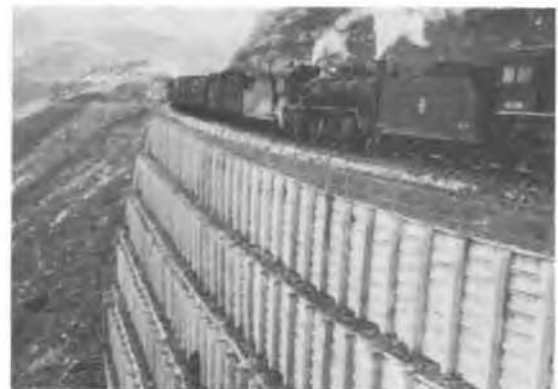
Fig.2 Photograph of the Shanxi Retaining Wall
