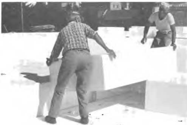
Fig. 3: Building with blocks of expanded polystyrene. The blocks are interlocked by using a staggered joint pattern. Double sided timber fasteners (e.g. Bulldog Ø 117 mm) shall prevent sliding on the underlying layer. (Photo: Refsdal)
