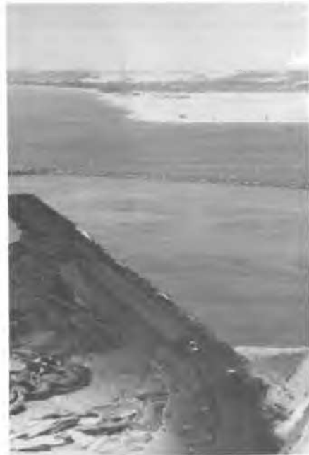
Fig.7: Construction of the dam.
