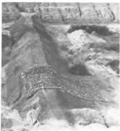
FIGURE 5b Filter dam with emergency spillway
