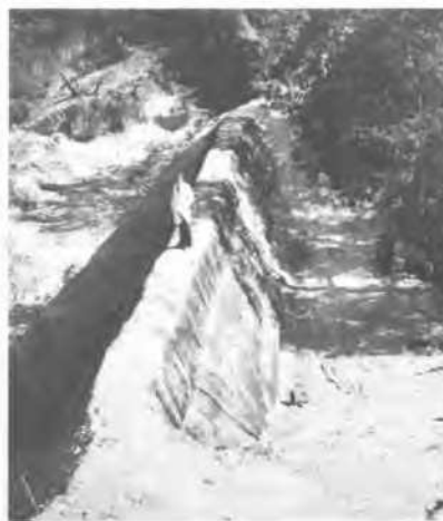
FIGURE 6b Completed geofabric-reinforced dam
