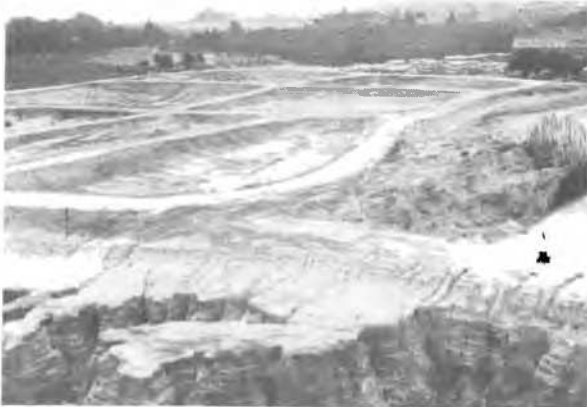
FIGURE 1b Abandoned, badly eroded tailings dam provided with crest and dividing walls.
