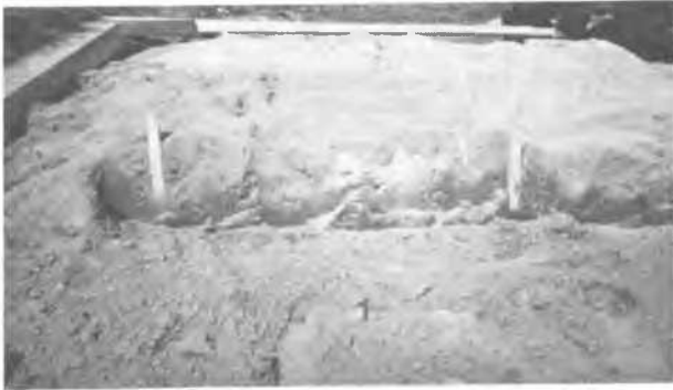
Fig. 2 A section through the soil/bentonite bed after 8 passes with a wheelless cultivator. Note the lenses of pure bentonite.
