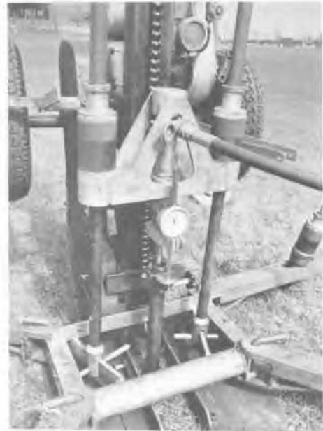
Fig. 6 The movable point is pushed down by a system of inner rods and the settlement of the point is measured on a dial gauge.
