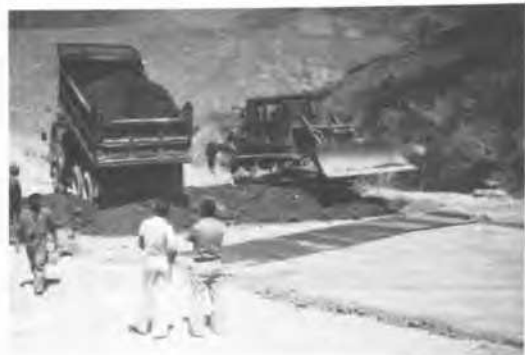
Fig. 4. - Embankment compaction on the flat jack
