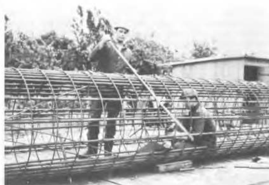
Fig. 1 Reinforcement cage of a large bored pile, diameter 150 cm
