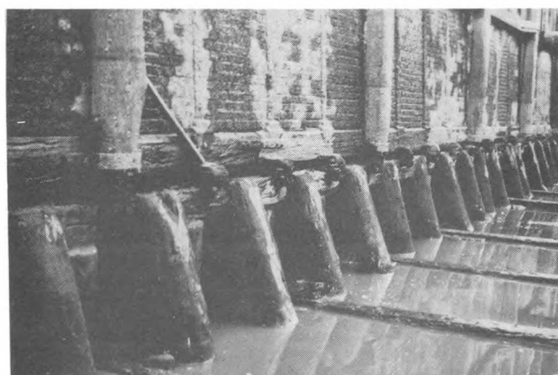
Fig. 6: Foundation of a sluise
