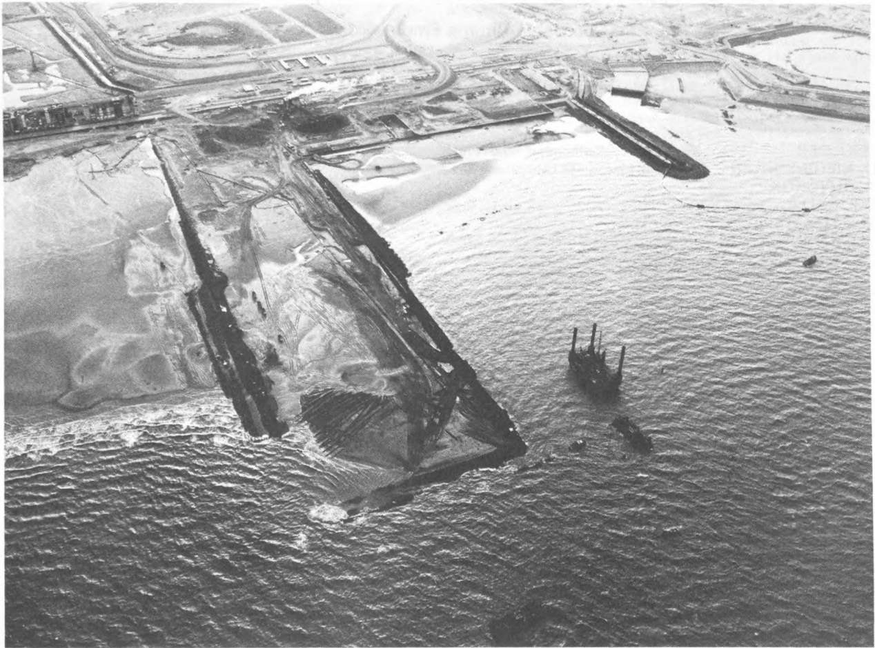
Figure 1. Sandasphalt protection dikes around a hydraulic fill for a wave breaker in the Northsea.
