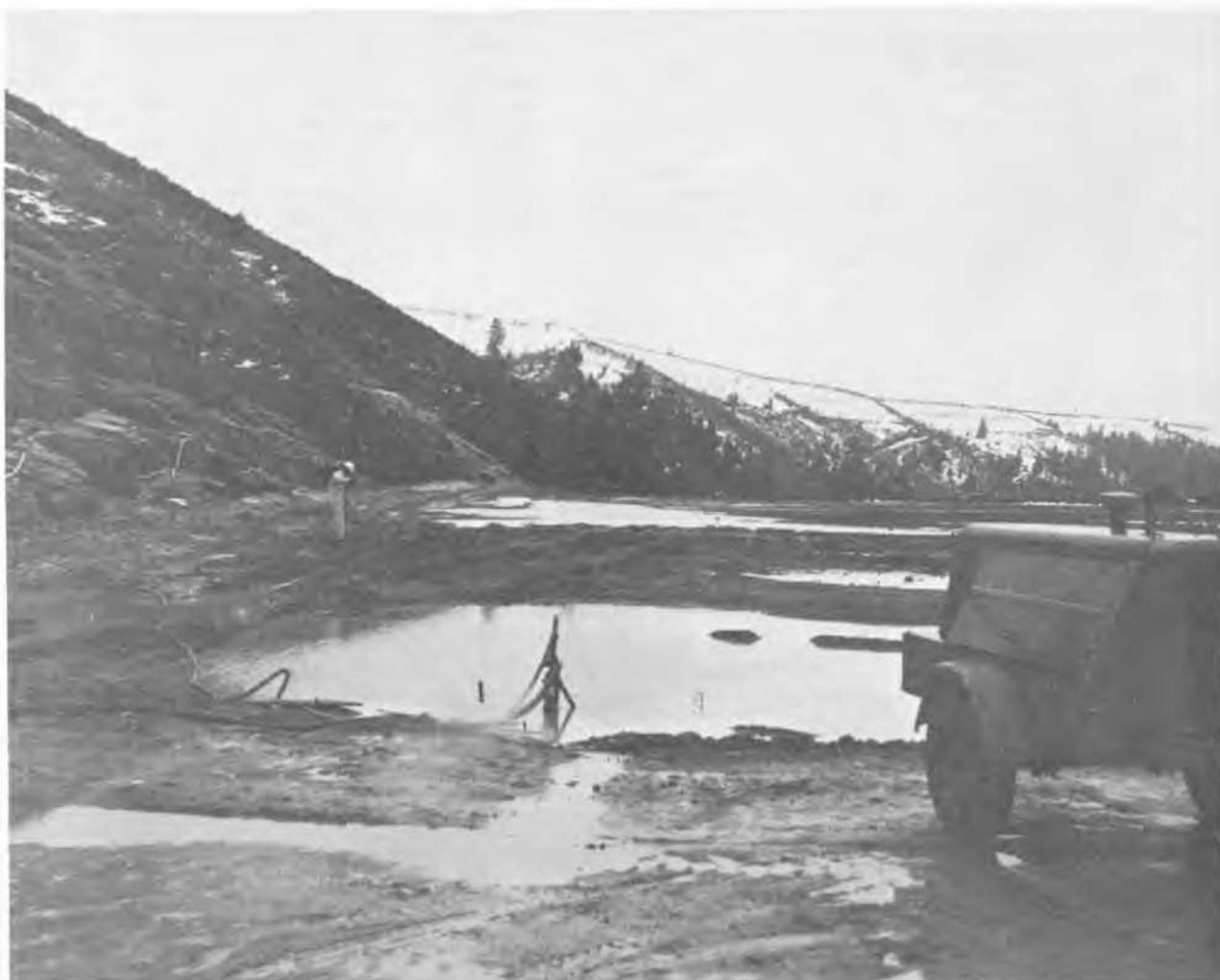
Fig. 11 Photograph of Water Ponded on Fill on Left Side of Embankment on May 7, 1975
