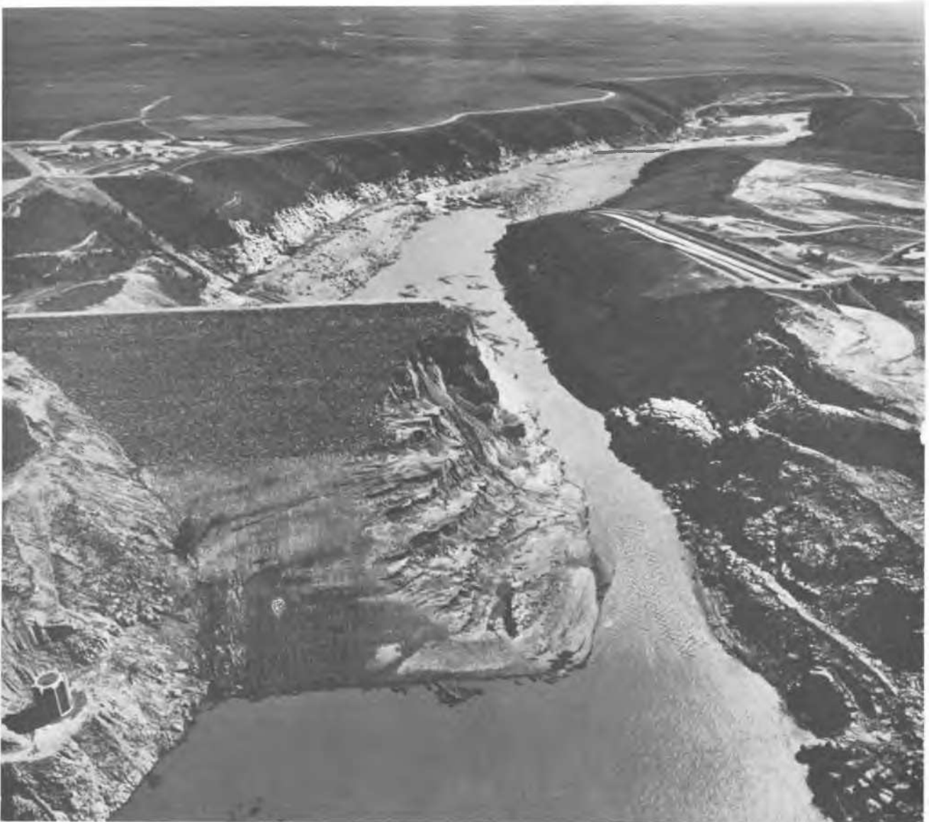
Fig. 4 View of Teton Dam After Failure
