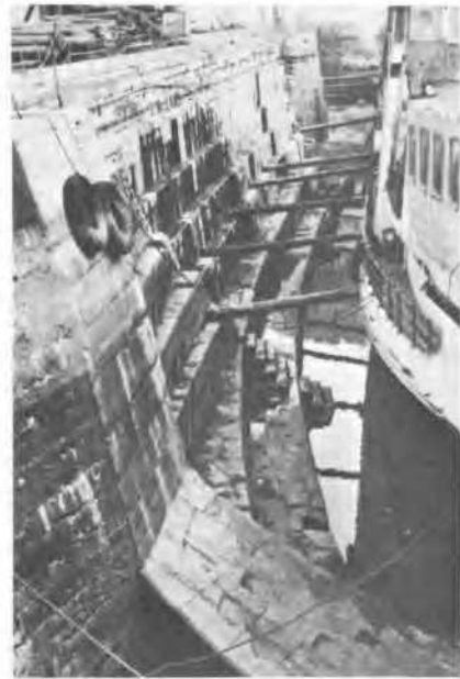
FIG. 2 - Present view of the once repaired corner.
