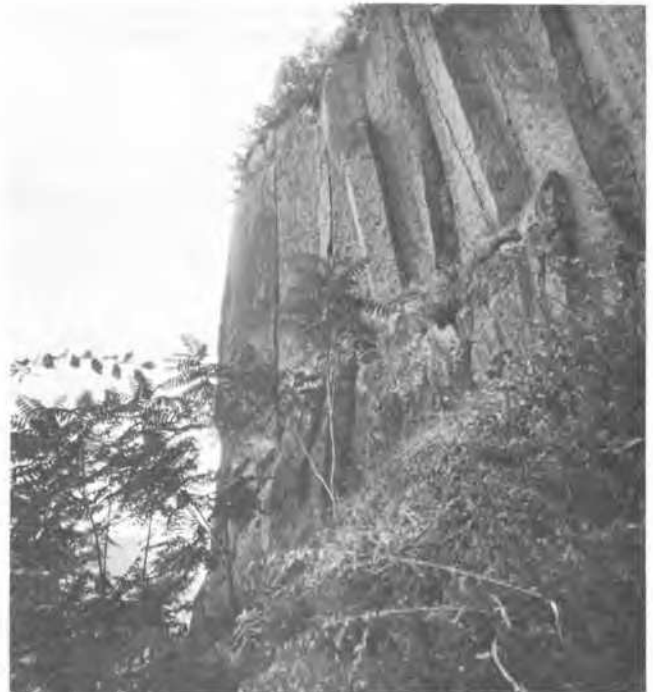
Fig. 7 - "Column" fracturing of a spur and "step-like" configuration of border areas
