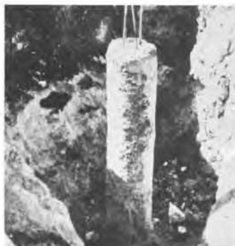
Fig. 1 Exposed typical Micropile.
