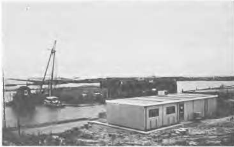
Figure 2 View of the test location
