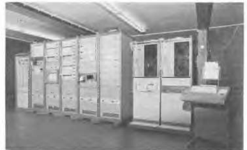
Figure 5 Interior of control room with function generators, analogue recorders, amplifiers, mag tape units and computer
