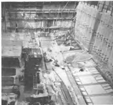
Fig. 8 Preparation of the cells in the site
