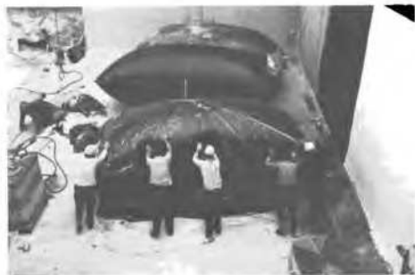
Fig. 7 Trial filling of the cushions by means of air pressure
