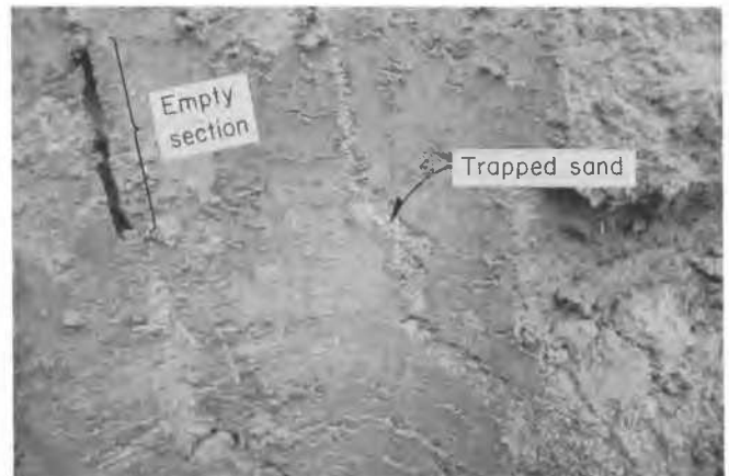
Fig 4. A front view of the cracks at the open pit
